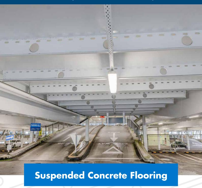
A high precision, concrete composite floor with integrated, cold-formed, pre-galvanised steel joists for superior strength and accuracy.
